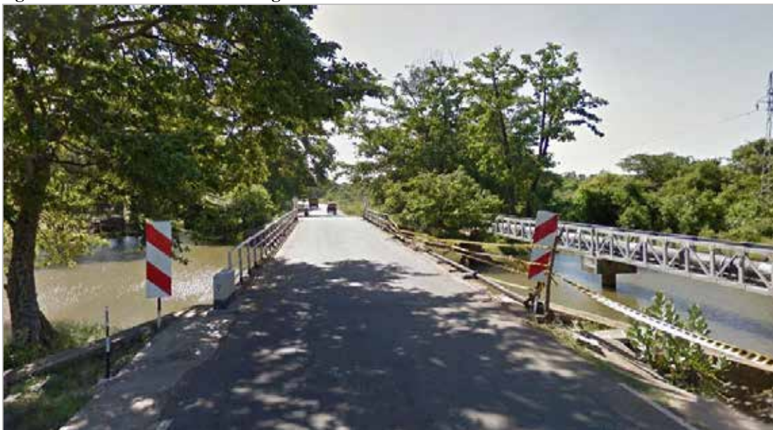
Figure 6.22 Gallella Narrow Bridge
