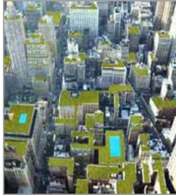
Figure 6.25: Green cover on roof
